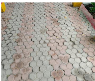
Paving stone installed in campus
