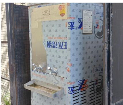
Push Taps In Water Cooler
