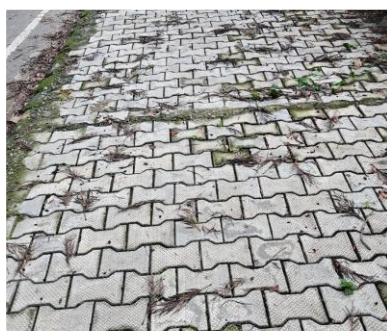
Paving Stone Installed In Campus
