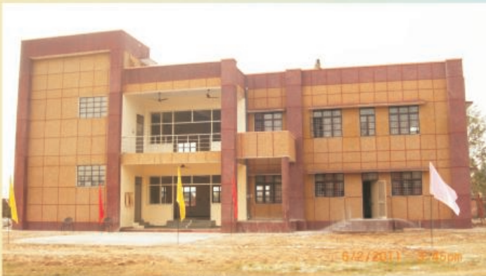
newly Constructed FET Canteen
